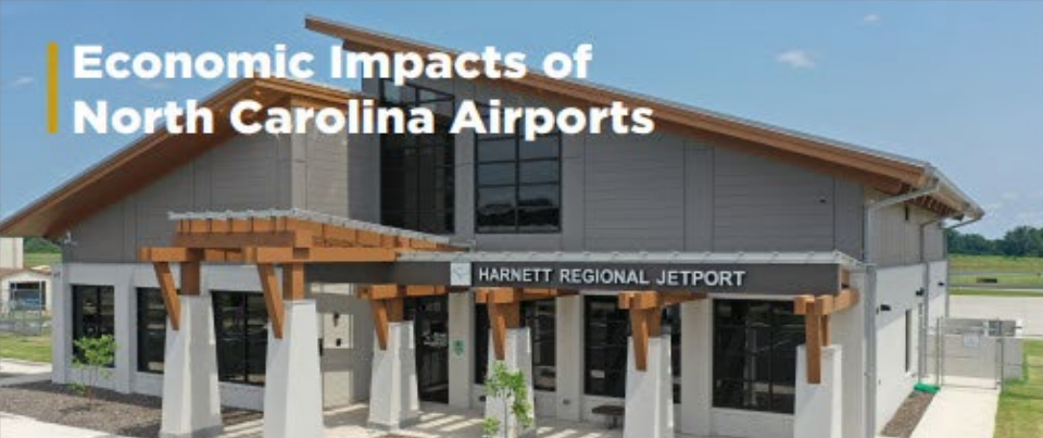
Harnett Regional Jetport unveiled its new 7,000-square-foot state-of-the-art terminal building in June 2024. It provides a modern, comfortable, convenient space for travelers and crew.
