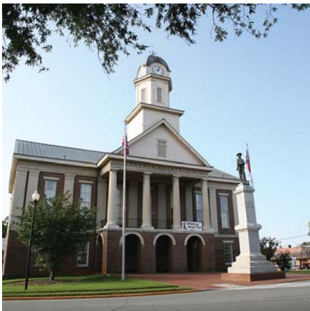
The courthouse in October 2009, prior to the beginning of renovations.
